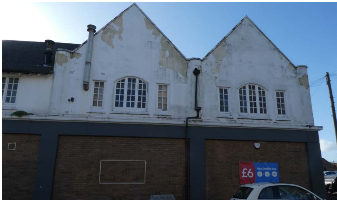
The current extended Co-op stores at Forest Town, February 2018
