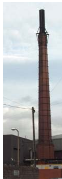
Figure 6: The circular brick chimney within the site
