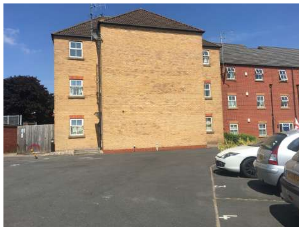
Figure 4.7 Poor relationship (building & street)
