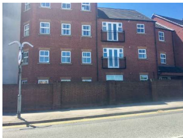
Figure 4.16 Poor relationship between building and street
