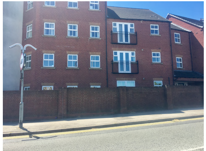
Figure 4.17 Poor relationship between building and street
