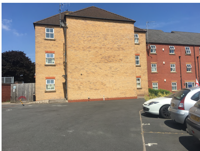
Figure 4.7 Poor relationship between building and street
