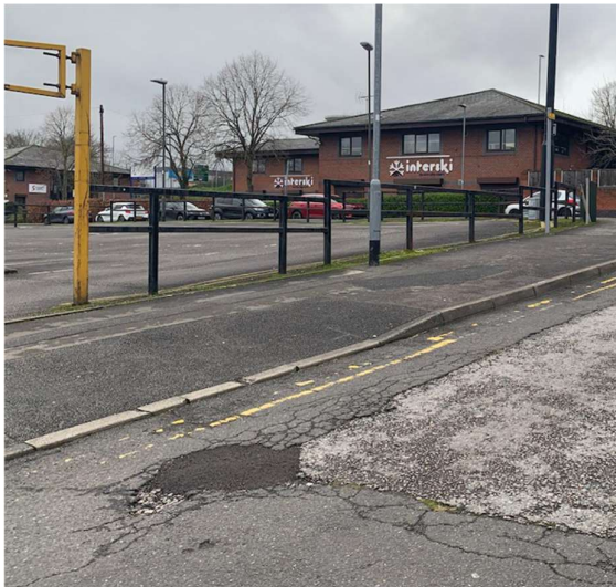
View of the Site, facing northwest
