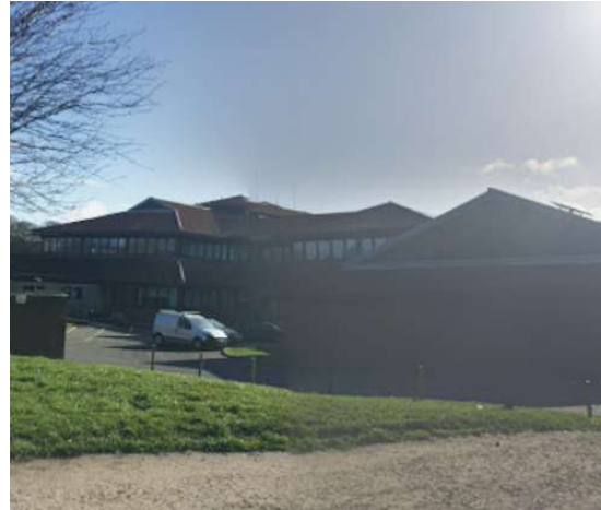
Site and surroundings
