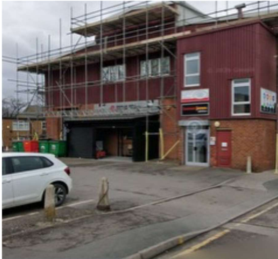
View of the Site
