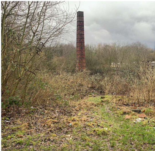
View of the chimney
