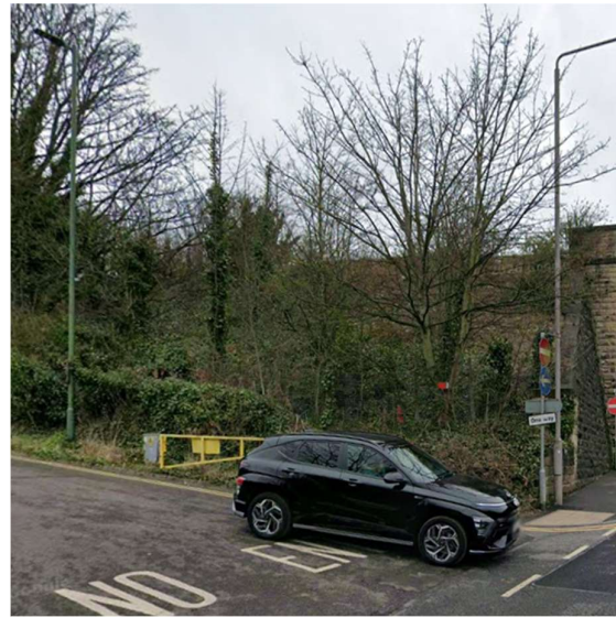
View of viaduct from the existing exit from the Site
