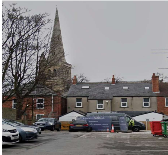
View of Gll church (1215129) and NDA terrace (MNT28677) from the Site
