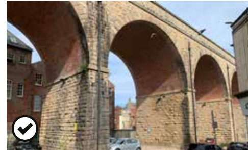
Railway Viaduct - built using local stone
