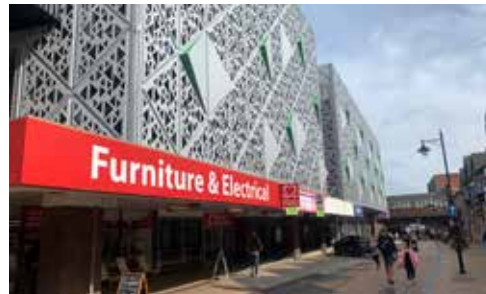
Walkden Street - public realm enhancement opportunity
