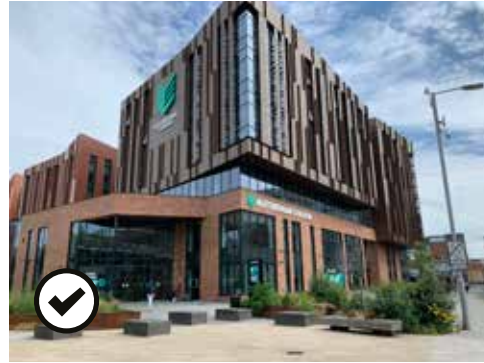
Tonally appropriate brick and cladding
