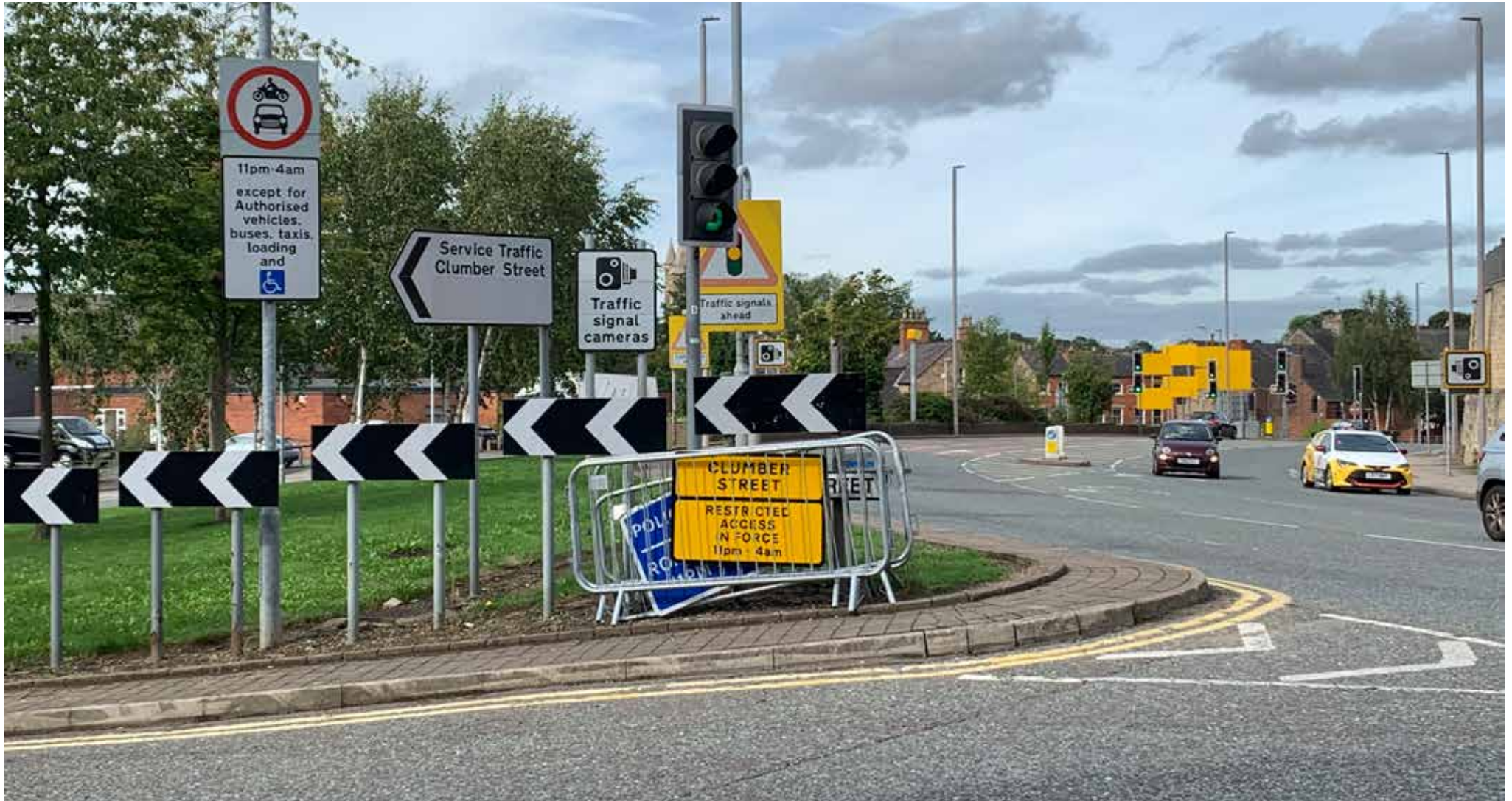
Excessive signage and street clutter should be removed
