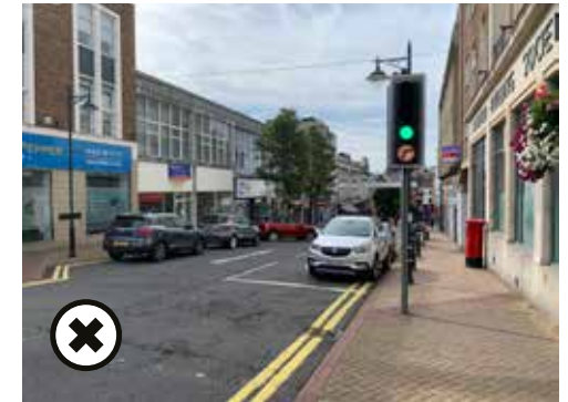
Large bright yellow lines should not be used in the town centre
