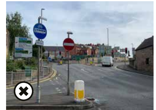
Excessive signage and street clutter should be removed
