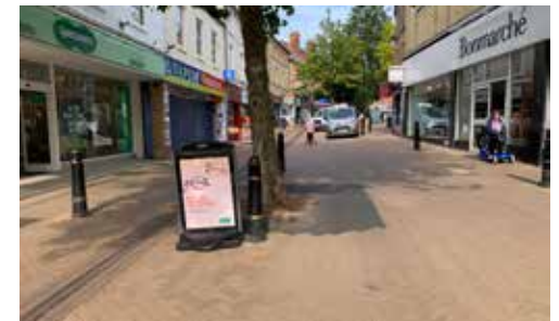
Keep a stock of materials to avoid patching with tarmac
