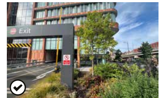
Landscaped car park entrance
