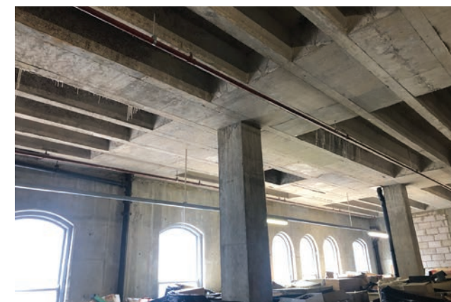
Figure 1.18: Modern structure behind the retained facade
