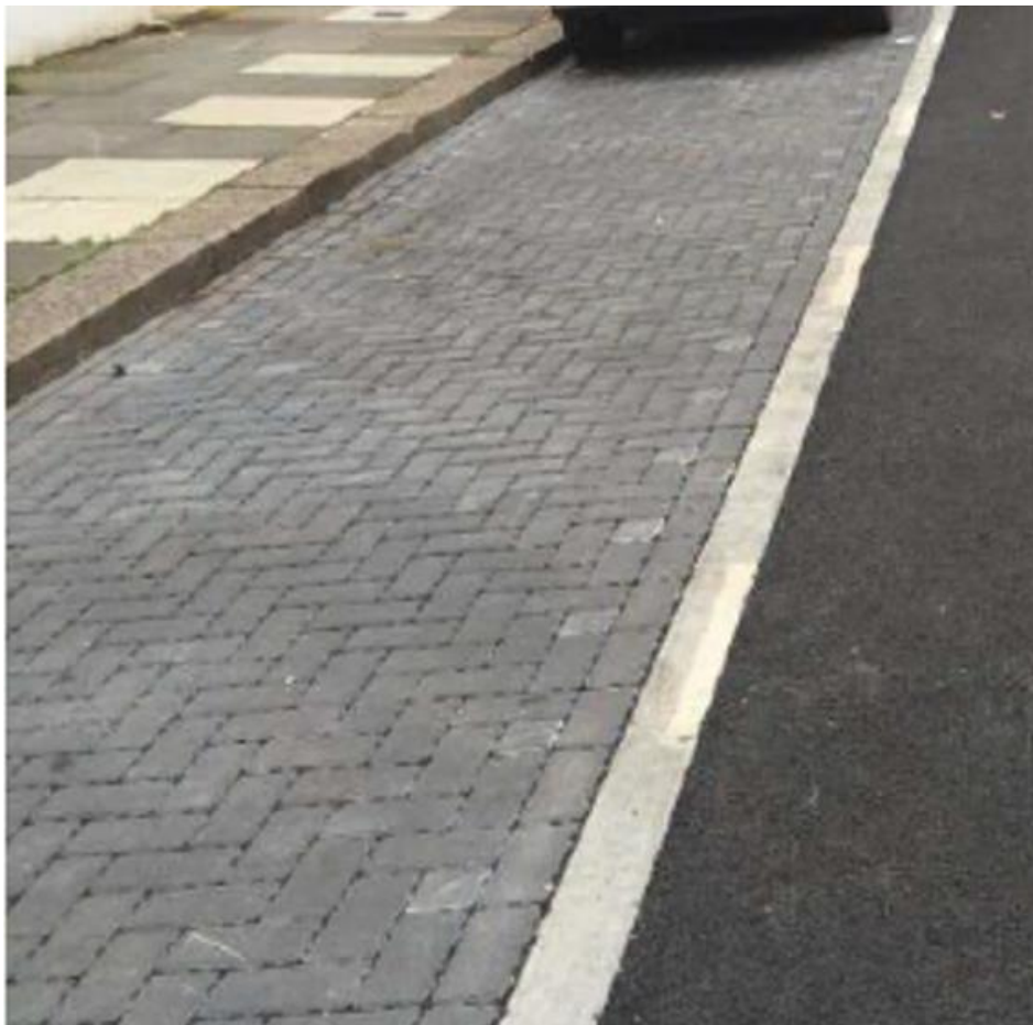
Photograph 5: Permeable paving
