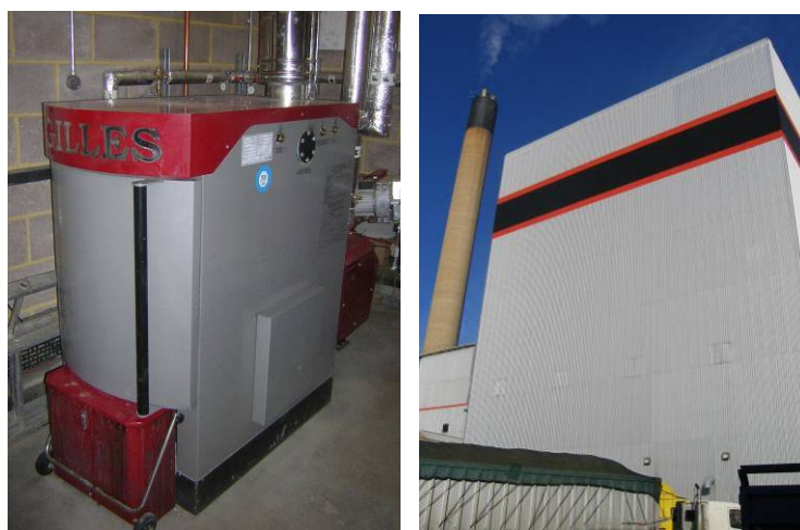
Left: Heat-only biomass boiler at Chilterns Burial site. Right: Biomass combined heat and power station at Slough
