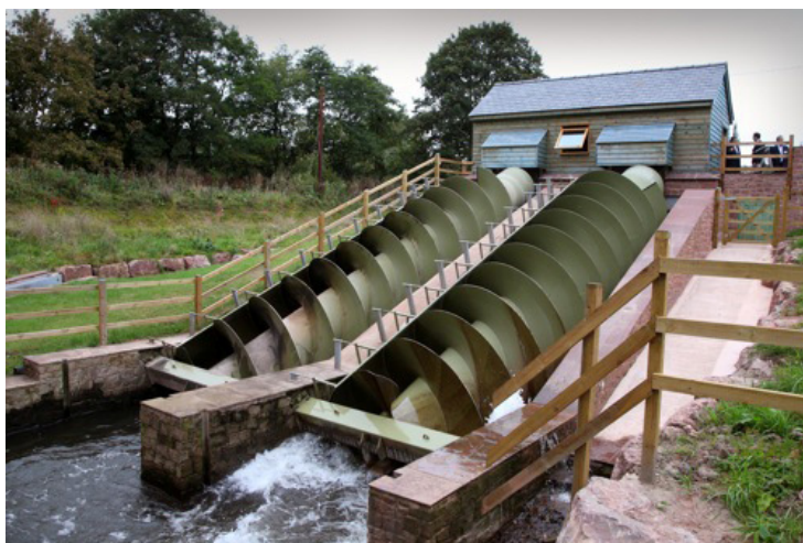
Osbaston 150kW hydropower scheme and fish pass on the River Monnow in Monmouthshire, opened 2009. [Source: www.aberdareonline.co.uk ]
