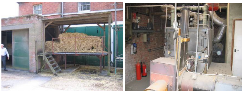
Straw bale combustion boiler providing heat to local buildings
