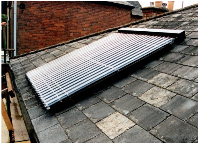
Solar thermal panel (evacuated tube system) [Source: www.cse.org.uk ]
