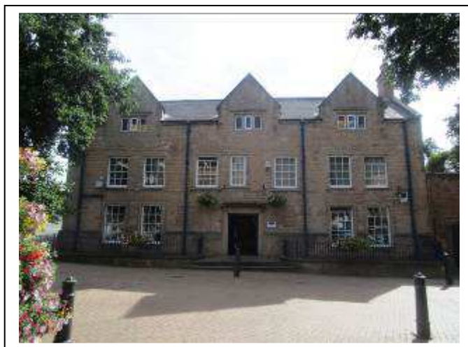
Post-mediaeval building, West Gate.
