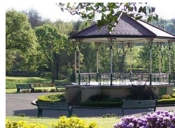
Bandstand refurbishment - link to play
