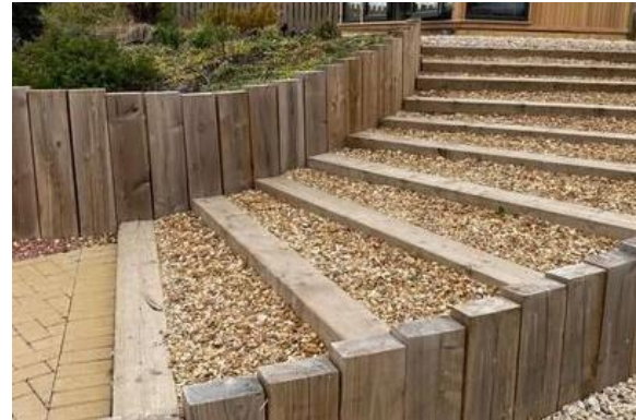
Access to play area in retaining wall
