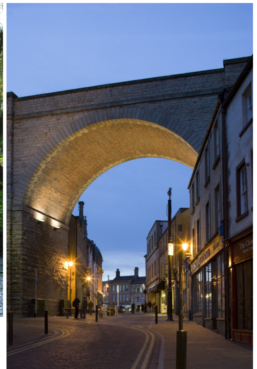
The Railway Viaduct
