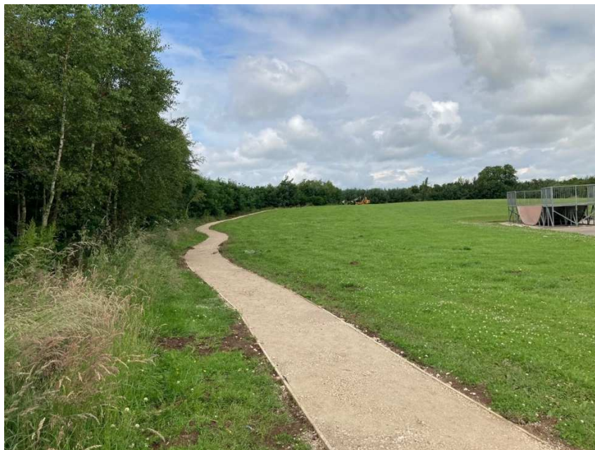
Photograph 4 – Crushed stone footpath to replace grass desire line path – Bull Farm, Mansfield
