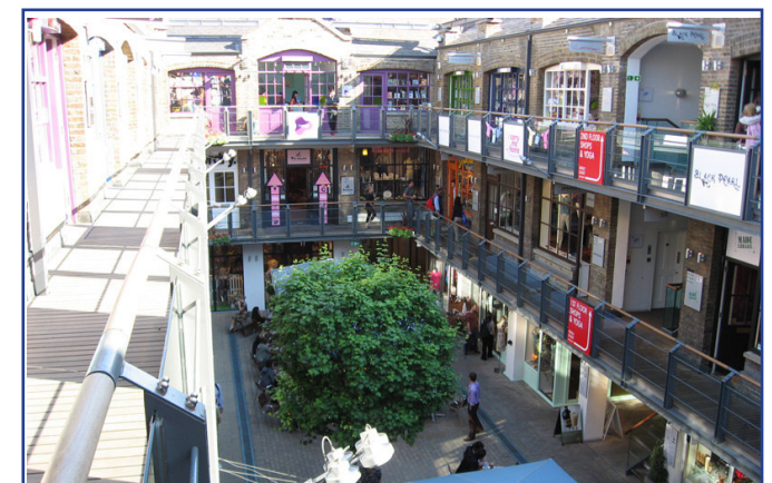
Kingly Court, Regent Street, London. An good example of the re-use and redevelopment of former industrial areas
