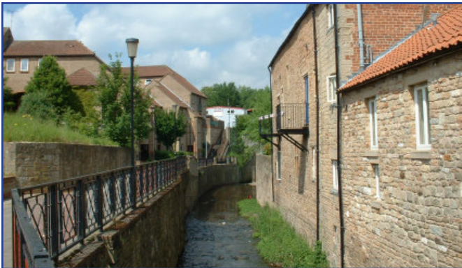
View looking north with adjacent historic buildings to east
