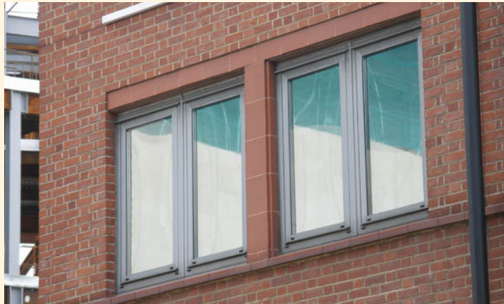
A modern interpretation of the traditional grouping of windows in an elevation, imparting a rhythm to the facade and avoiding the repetitive nature of modern facades. The tendency to have over-deep spandrels between the windows on each floor is addressed to some extent by the use of string courses.
