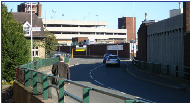
Four Seasons Centre - Southern elevation to Quaker Way
