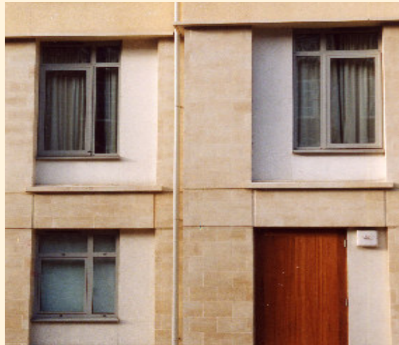
Elevations can be designed to increase scale and modelling in prominent urban locations through the subtle recession and projection of elements.
