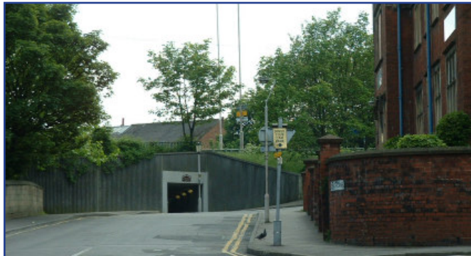
St Peter's Way, Church Lane junction
