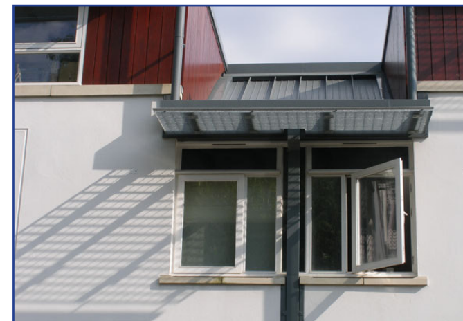
The interplay of a rendered elevation with a sunscreen can produce a lively facade. The well proportioned windows are separated by a metal half recessed downpipe, fully integrated into the elevational design.
