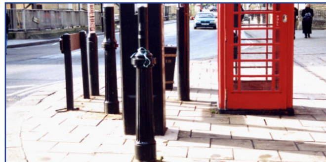
Eliminating clutter - a key objective in placing street furniture
