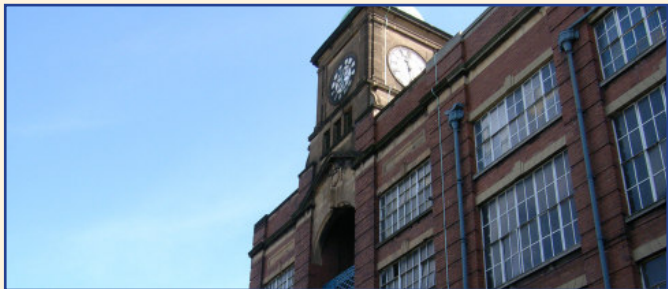
Bath Lane Works
