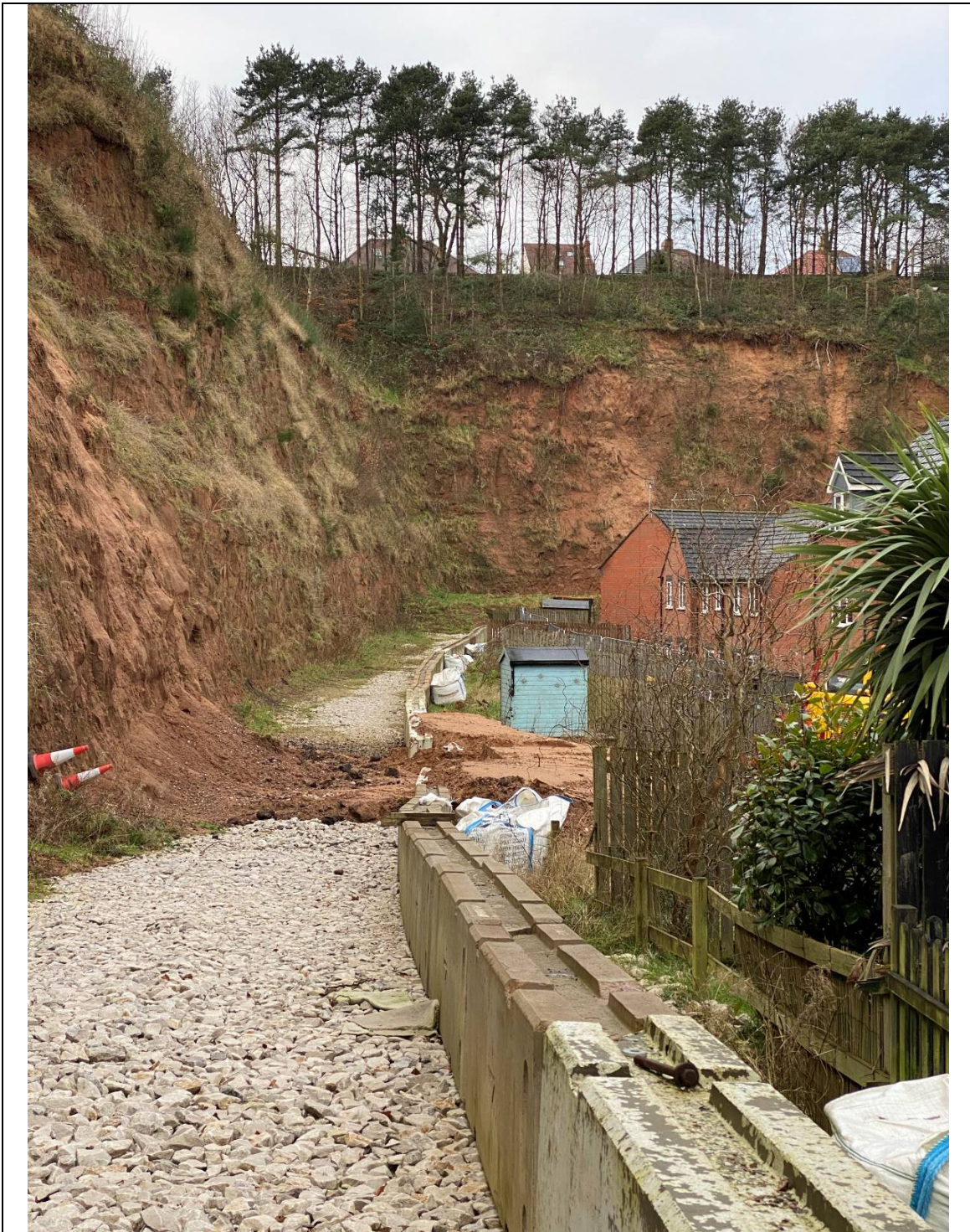
Photograph 1: Looking along the southern flank of the quarry to the south west corner. Note, the small amount ( \sim 3\text{m}^3 ) of slope debris at the toe of the slope, contained within the rock trap. The debris has amassed following the clear up operations from a recent failure on the night of 23 rd of December 2020 and originates from the residual material at the crest of the recent failure scar (Image taken on 05/01/2021)
