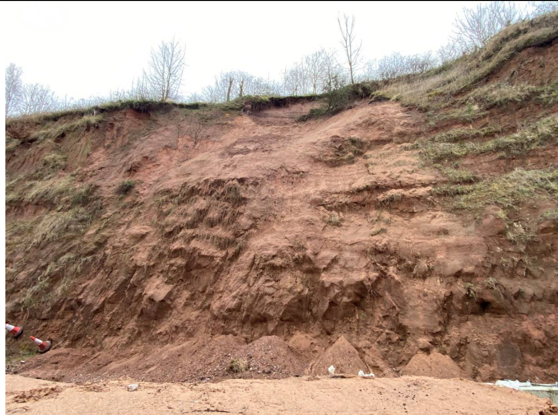
Photograph 2: Previous failure scars which appears to be partially saturated in surface water run-off from recent rain and snowfall. Note the small amount of failure debris ( \sim 3\text{m}^3 ) at the toe of the slope which has amassed since the clear up operation of a recent failure on the 23 rd of December 2020. (Image taken on 05/01/2021)
