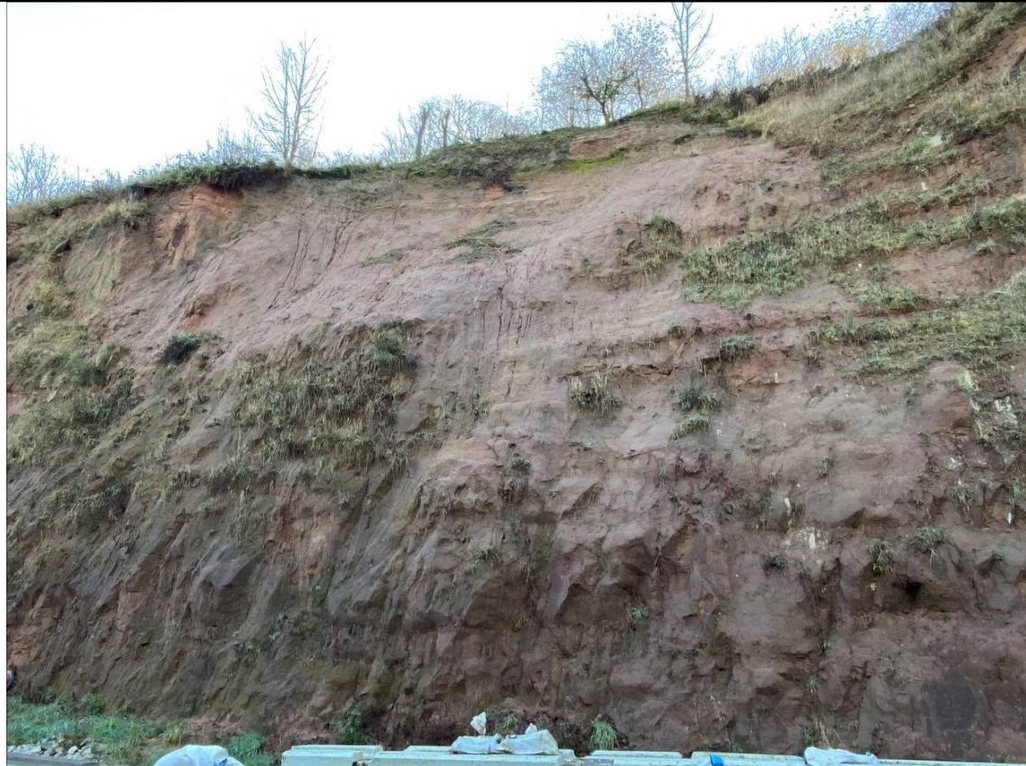
Photograph 2: Previous failure scar which appears to be partially saturated in surface water run-off (Image taken on 15/12/2020)
