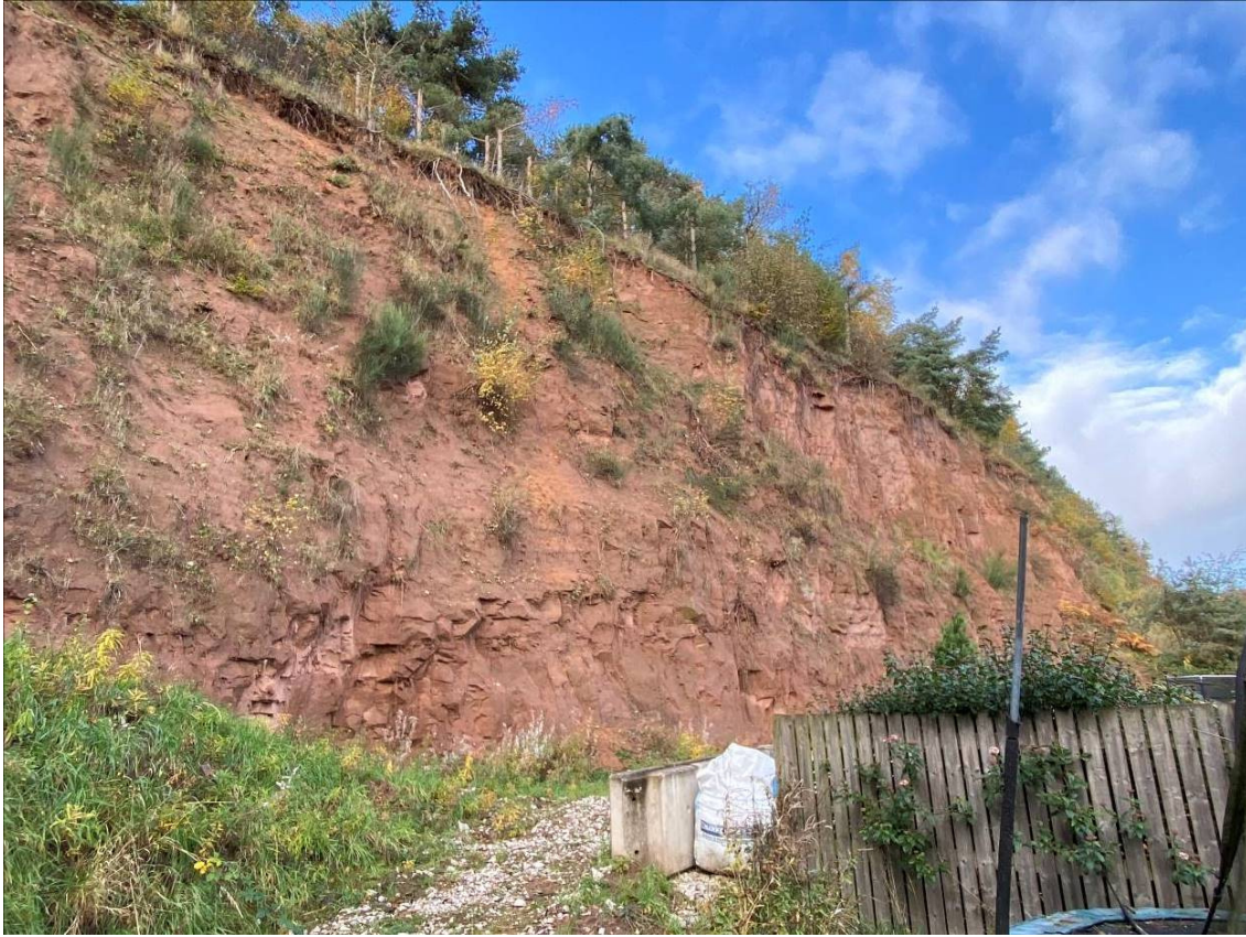
Photograph 4: Looking at the western flank. Note towards the centre of picture the orange streak of sand being washed down the cliff face from what appears to be the soil crust at the crest of the cliff. This is creating talus and sand mound at the toe of the cliff (Image taken on 03/11/2020).
