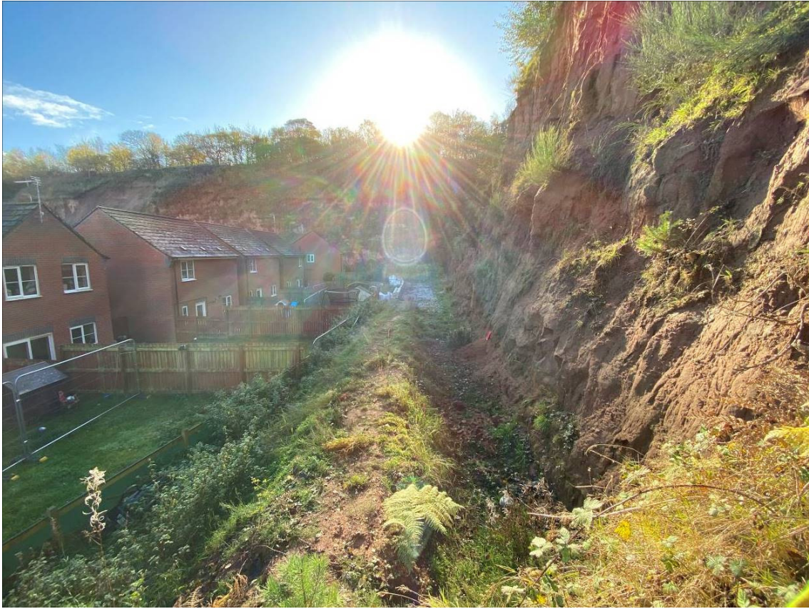
Photograph 5: Looking at the southern flank (background) and western flank (right-hand-side) with temporary earthwork bund and rock trap next to it (Image taken on 03/11/2020)
