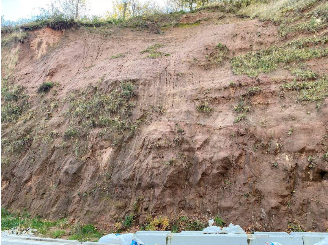
Photograph 2: Previous failure scar (Image taken on 03/11/2020)
