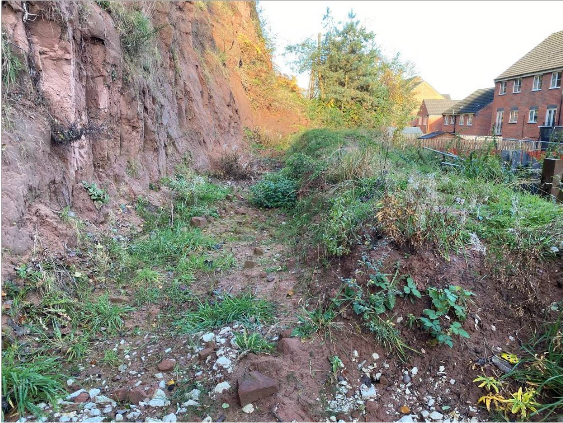
Photograph 6: Looking north to the end of Unit 8. The western flank is to the left-hand-side of the photograph with temporary earthwork bund and rock trap next to it. Note the scattering of small <30\text{cm}^3 unravelled sandstone blocks in the rock trap. (Image taken on 03/11/2020).
