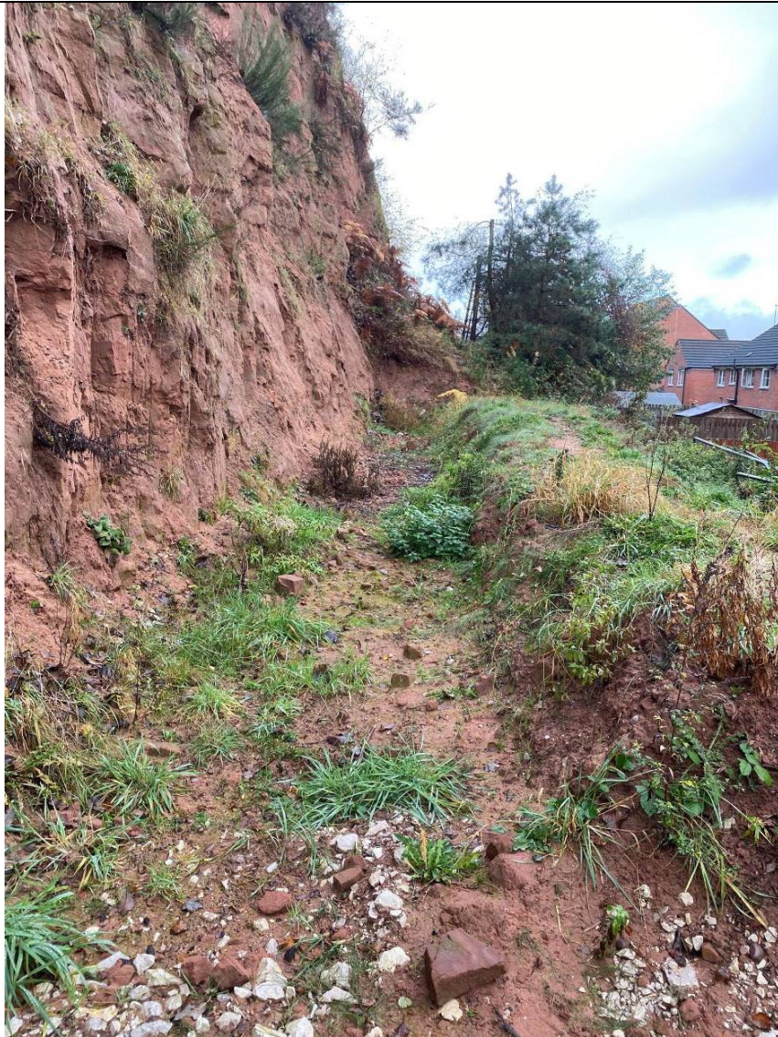
Photograph 6: Looking north to the end of Unit 8. (Image taken on 10/11/2020).
