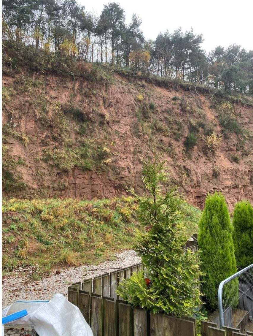
Photograph 3 : Looking west to the south west quarry corner (Image taken on 10/11/2020)
