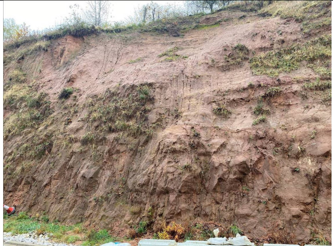
Photograph 2: Previous failure scar (Image taken on 10/11/2020)
