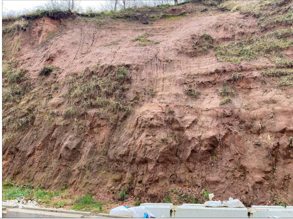
Photograph 2: Previous failure scar (Image taken on 17/11/2020)
