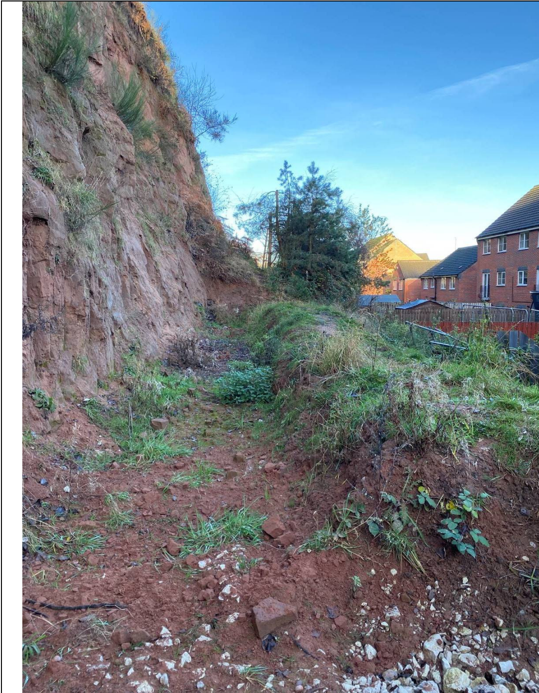
Photograph 6: Looking north to the end of Unit 8. Note the scattering of fresh soil debris in the foreground, originating from what appeared to be the overhanging soil crust at the crest of the cliff face. (Image taken on 01/12/2020).
