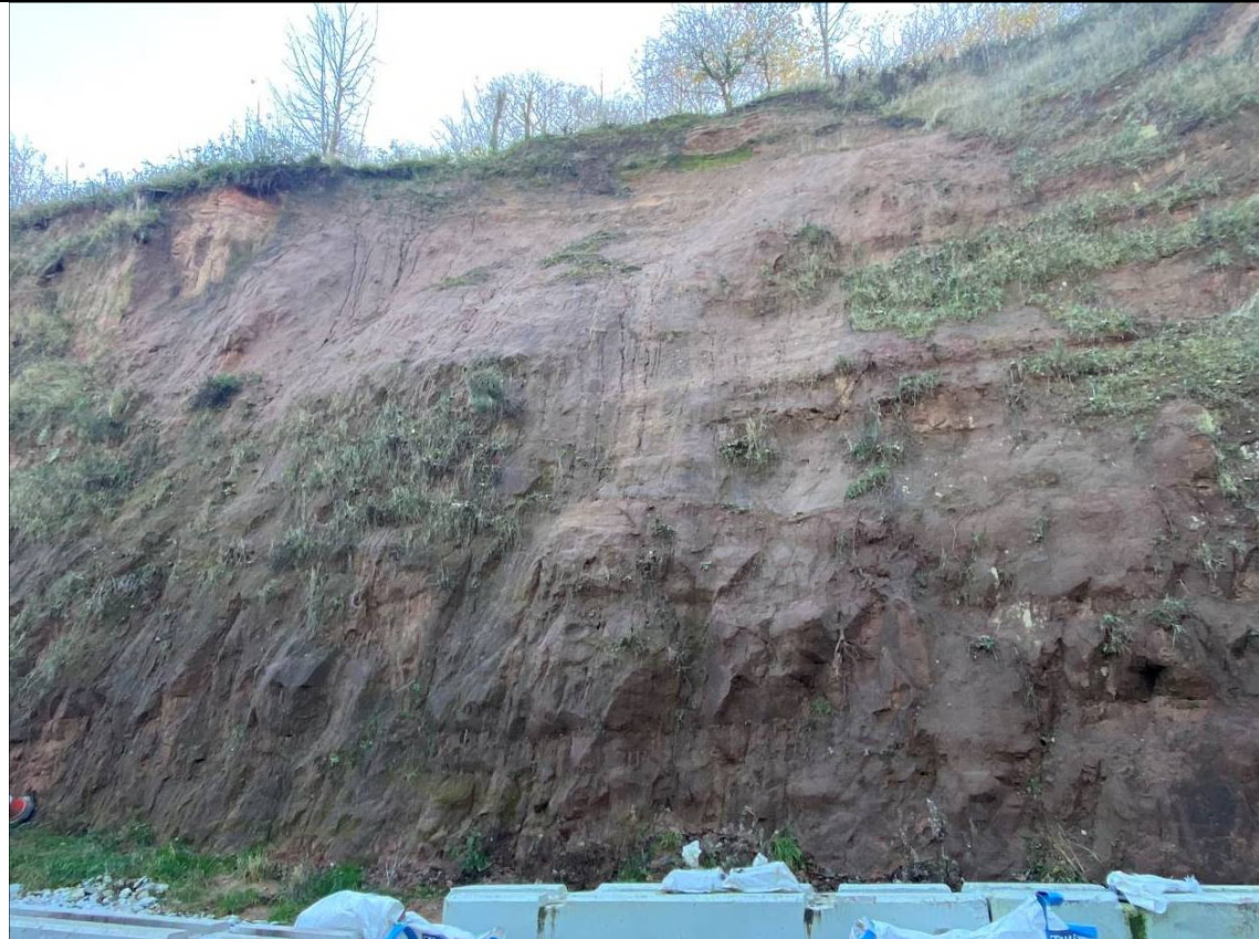
Photograph 2: Previous failure scar which appears to be partially saturated in surface water run-off (Image taken on 01/12/2020)
