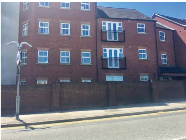
Figure 4.17 Poor relationship between building and street
