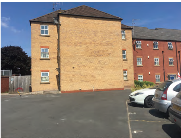
Figure 4.7 Poor relationship between building and street
