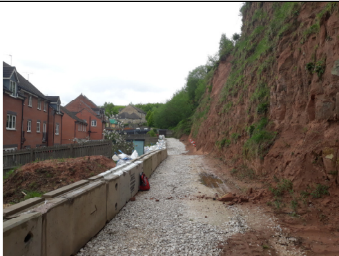
Photograph 6a and 6b: Small Ravel Failure Behind Unit 6 / 7 Boundary. (Images taken 30/04/2020).
