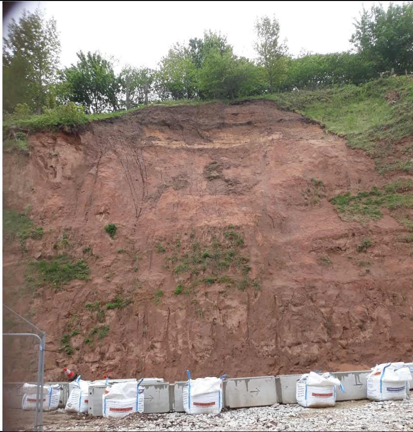
Photograph 2A: Previous failure scar (Image taken on 30/04/2020) with similar evidence of desiccation cracks and overhanging overburden/relic topsoil as that observed on 16/04/2020 inspection.
