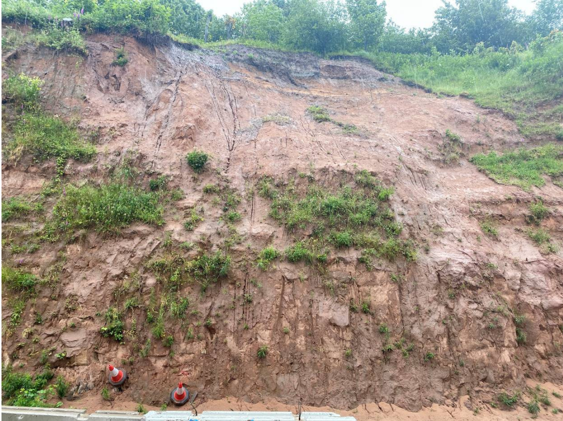
Photograph 2: Previous failure scar (Image taken on 18/06/2020)
