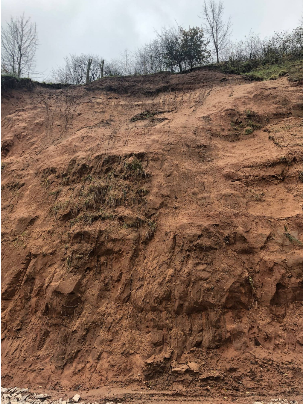
Photograph 2: Previous failure scar
