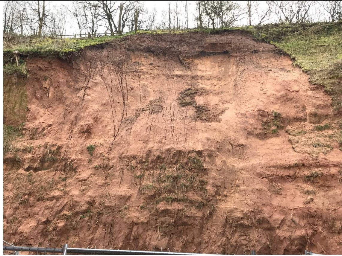
Photograph 2: Previous failure scar (Image taken on 18/02/2020)
