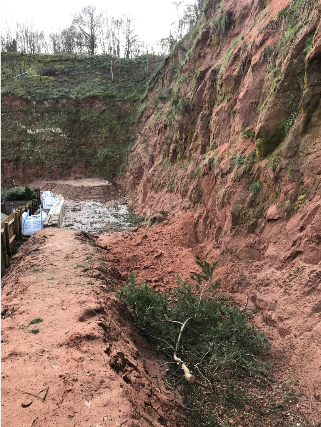
Photograph 5 : Looking at western flank and previous failure scar (Image taken on 18/02/2020)
