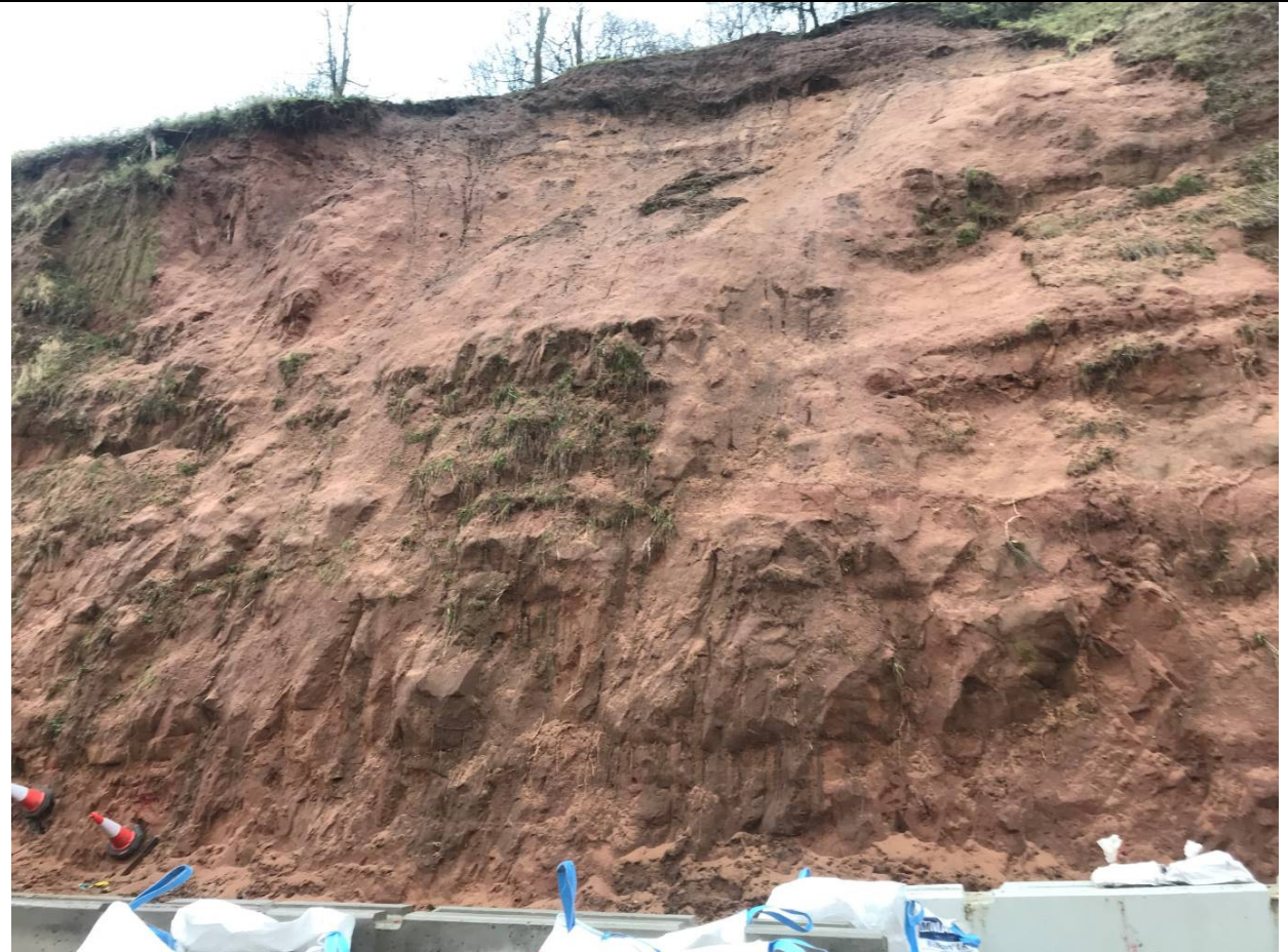
Photograph 2: Previous failure scar within the middle of Unit 9 (Image taken on 13/01/2020)
