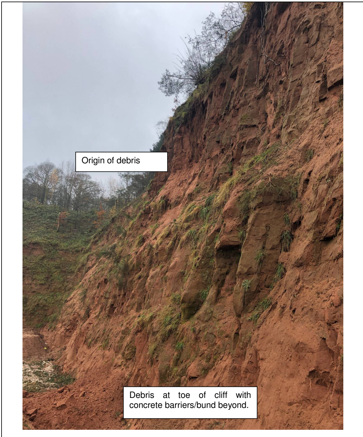
Photograph 1 : Location of small failure
