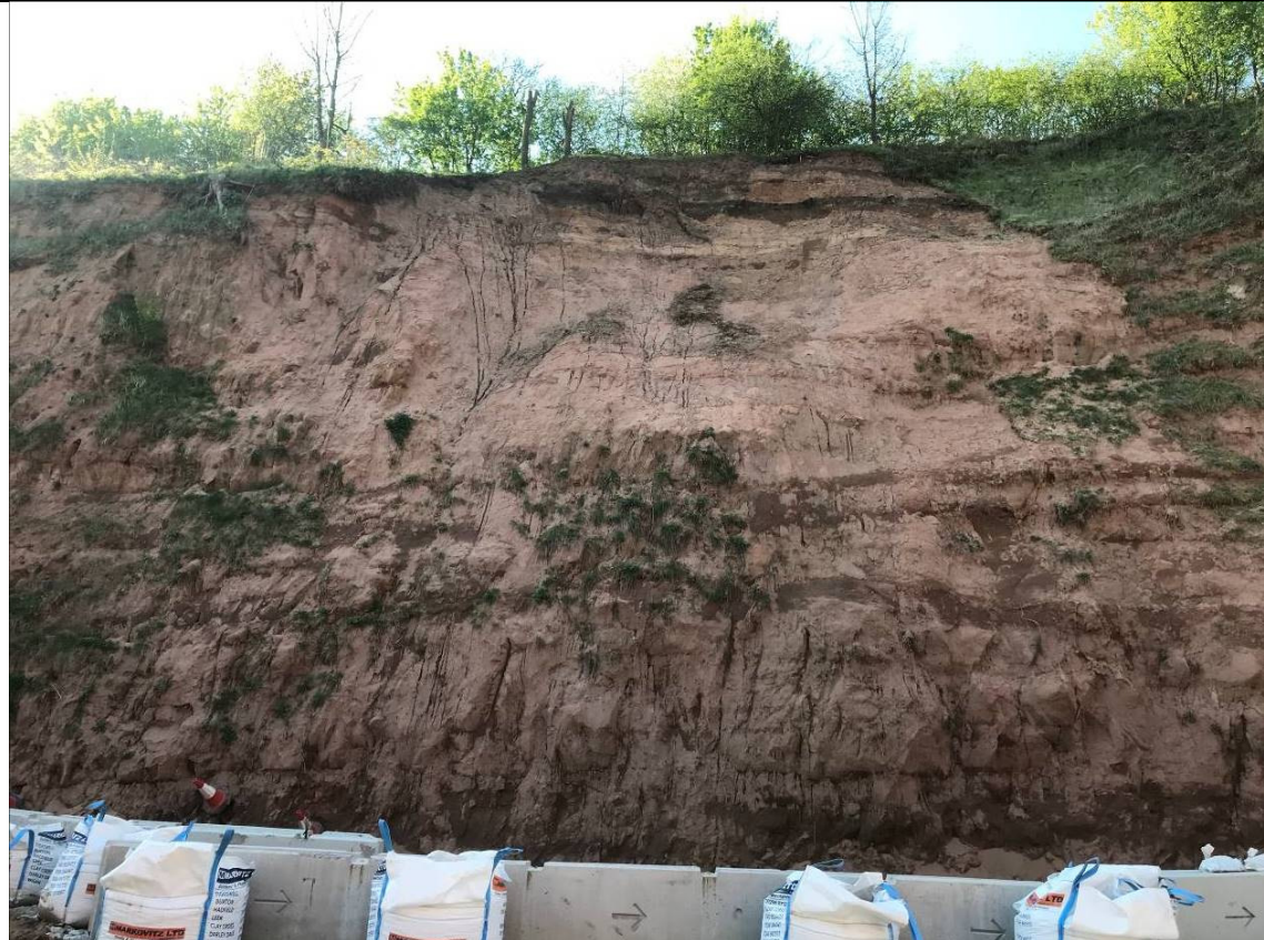
Photograph 2A: Previous failure scar (Image taken on 16/04/2020) with evidence of desiccation cracks and overhanging overburden/relic topsoil.
