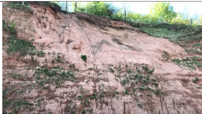
Photograph 2A: Previous failure scar (Image taken on 16/04/2020) with evidence of desiccation cracks and overhanging overburden/relic topsoil.
