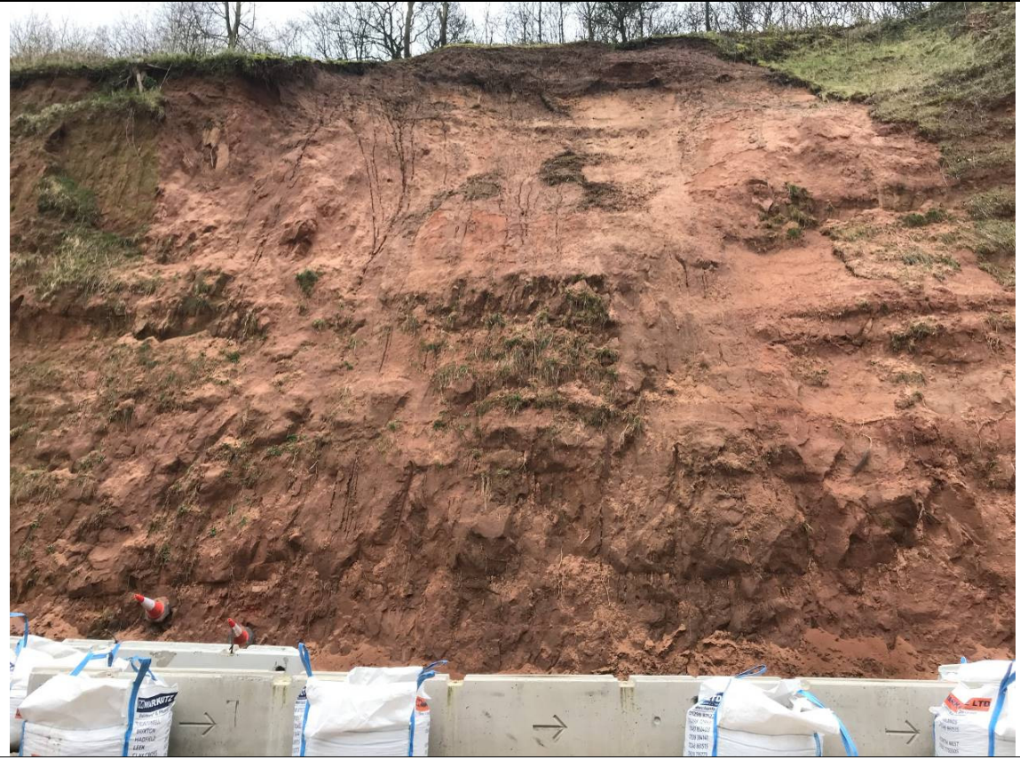
Photograph 2: Previous failure scar (Image taken on 05/03/2020)
