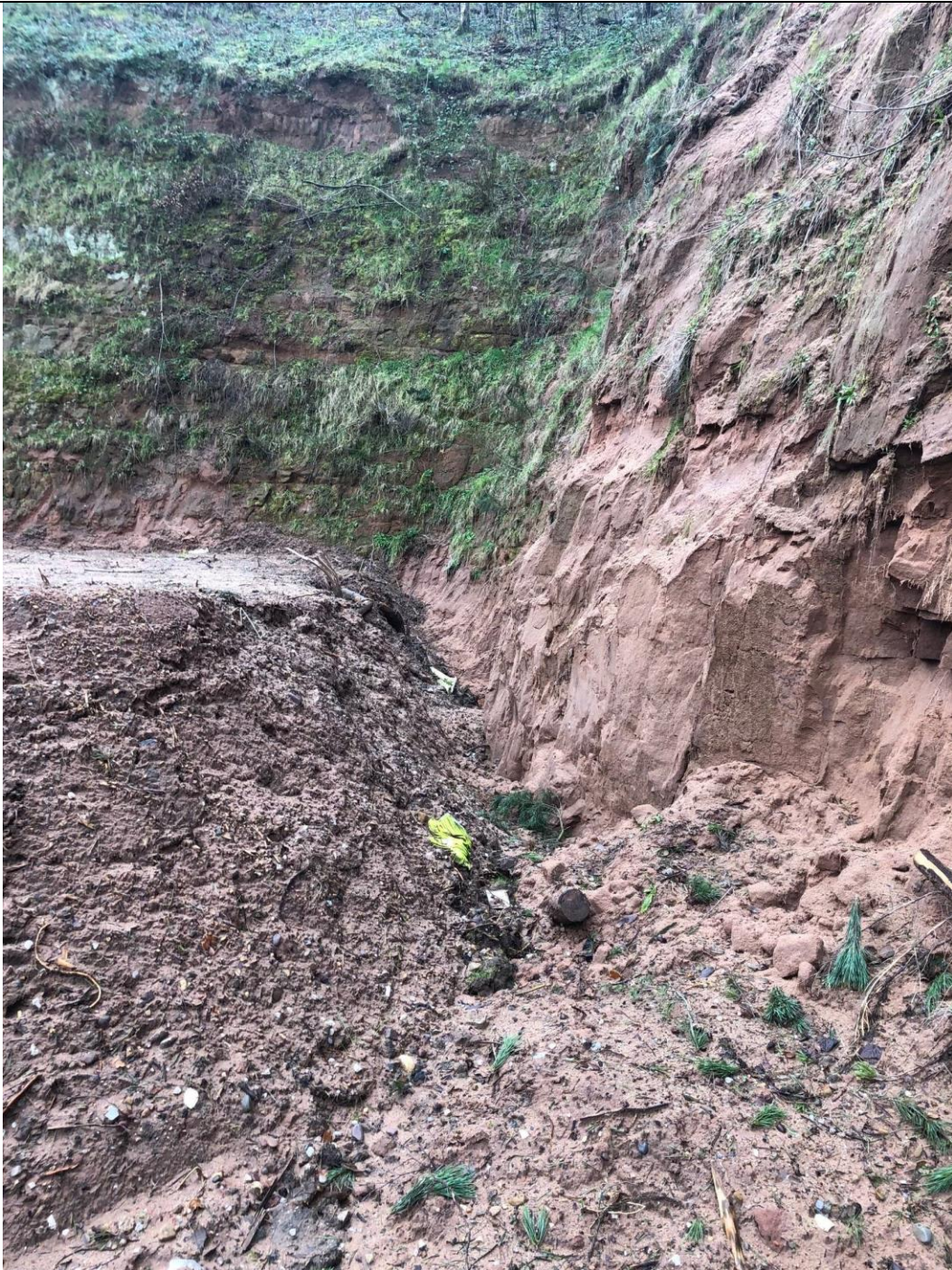
Photograph 3 : Rock trap between bund and quarry wall to rear of Plot 90 (Image taken on 30/01/2020)
