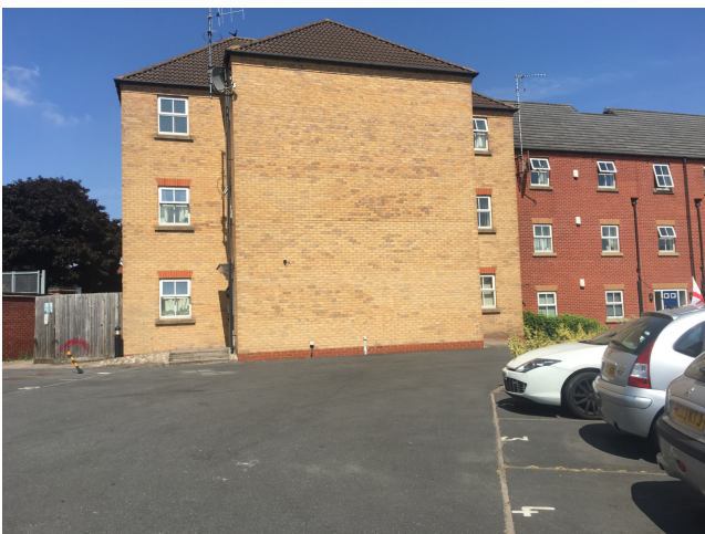
Figure 4.7 Poor relationship between building and street
