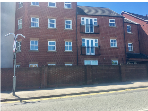
Figure 4.17 Poor relationship between building and street
