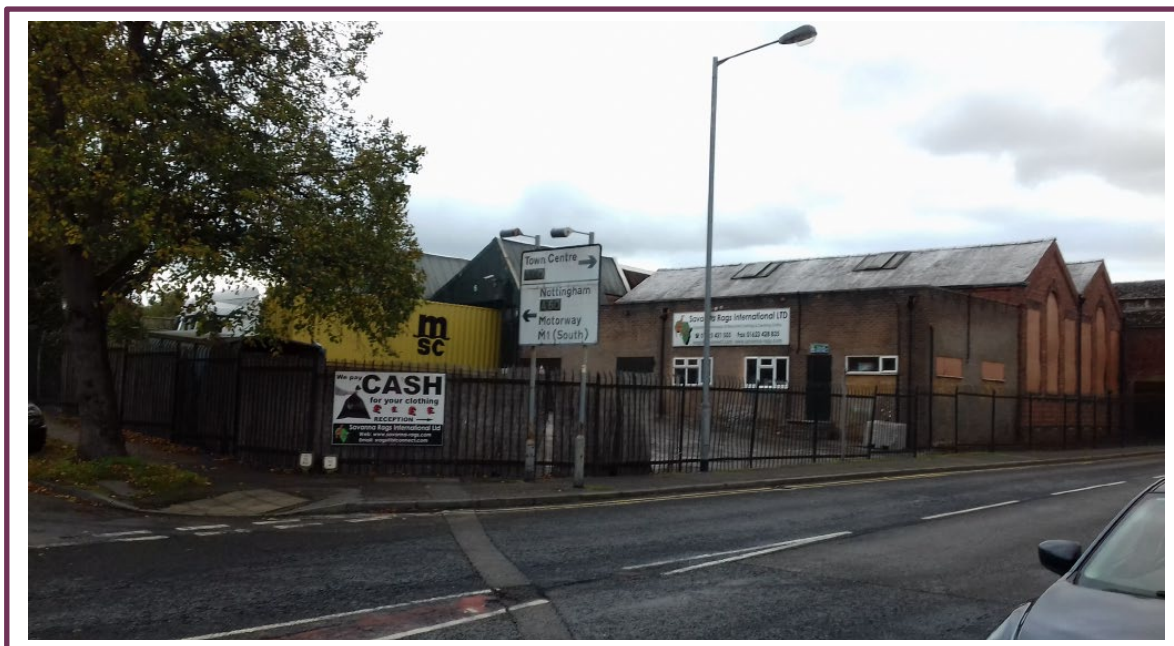
Photograph of existing employment unit taken from Forest Road.
