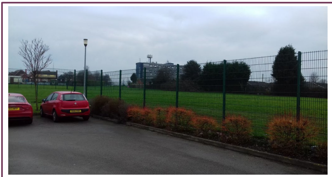
Photograph of northern side of the site looking south west.
