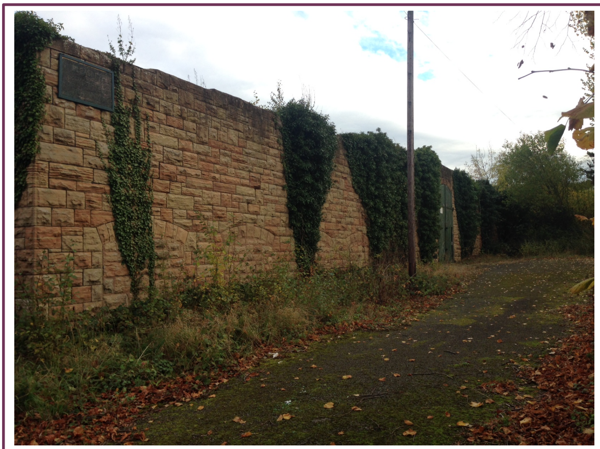
Photograph of existing structure on site from western edge looking south.
