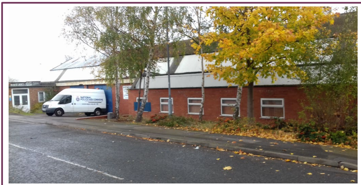
Photograph of southern elevation of existing building taken from Long Stoop Way.
