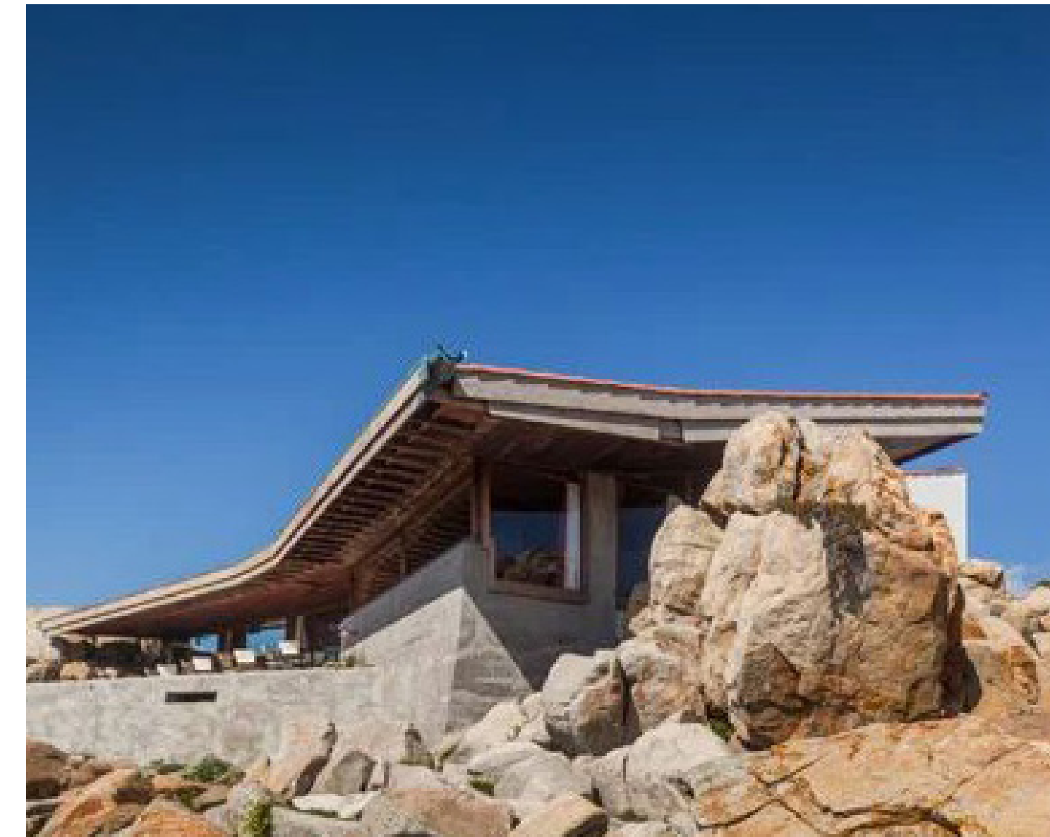
Stone base and timber roof
