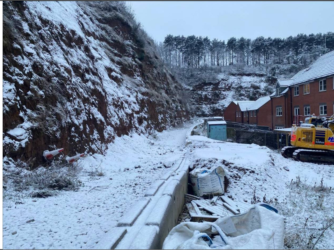
Photograph 1: Looking along the southern flank of the quarry to the south west corner. Note, the small amount ( <2\text{m}^3 ) of slope debris at the toe of the slope, contained within the rock trap. The debris amassed following the recent failure on the night of 23 rd of December 2020 and originates from the residual material at the crest of the recent failure scar (Image taken on 29/12/2020)
