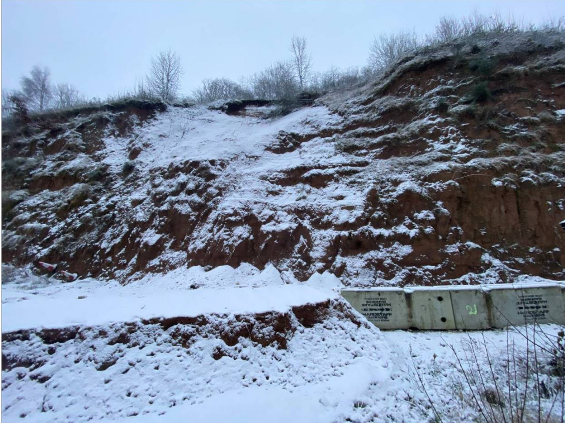
Photograph 2: Previous failure scars which appears to be partially saturated in surface water run-off from recent rain and snowfall. Note the small amount of failure debris ( <2\text{m}^3 ) at the toe of the slope which has amassed since the recent failure on the 23 rd of December 2020. (Image taken on 29/12/2020)
