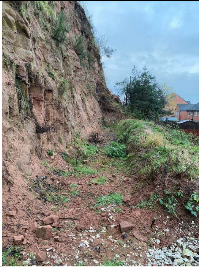
Photograph 6: Looking north to the end of Unit 8. Note the scattering of fresh soil and rock debris in the foreground, originating from what appeared to be just below the overhanging soil crust at the crest of the cliff face. (Image taken on 08/12/2020).
