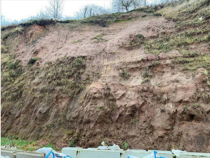
Photograph 2: Previous failure scar on which surface water run-off is apparent (Image taken on 08/12/2020)
