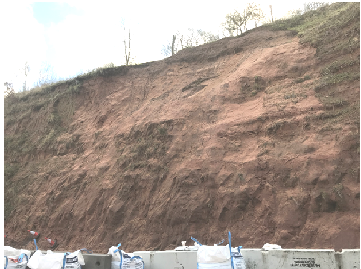
Photograph 2: Previous failure scar (Image taken on 23/12/2019)
