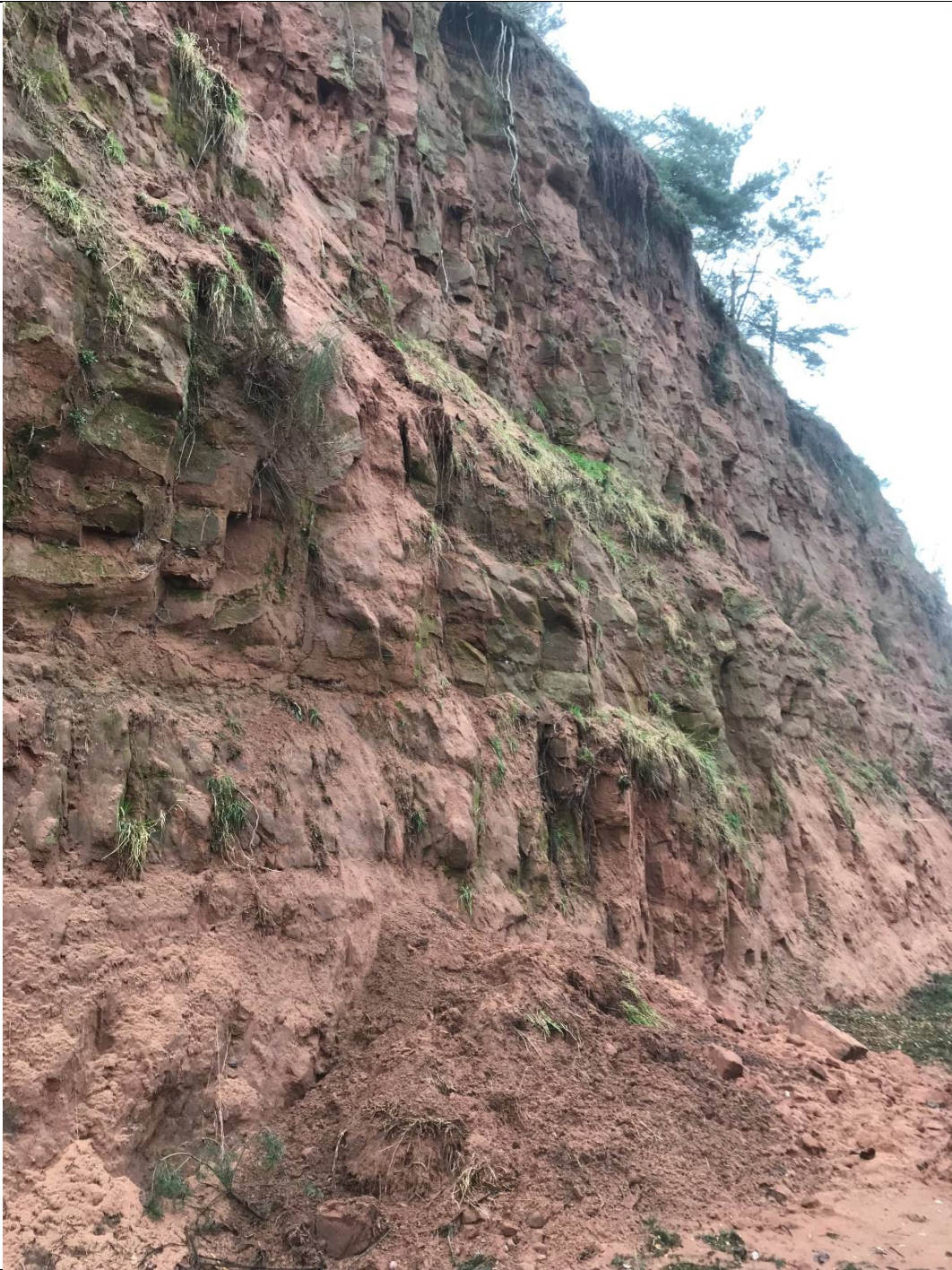
Photograph 5: Looking north to the end of Unit 8. Debris from small failure reported on the 24 th November 2019. Note two vegetation clumps, approx. 30cm 2 on top of the previous small failure (Image taken on 23/12/2019).
