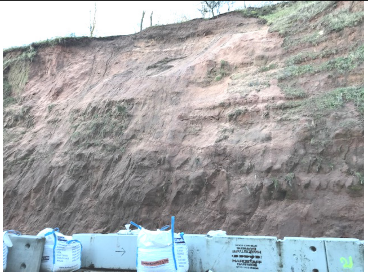
Photograph 2: Previous failure scar within the middle of Unit 9 (Image taken on 20/01/2020)
