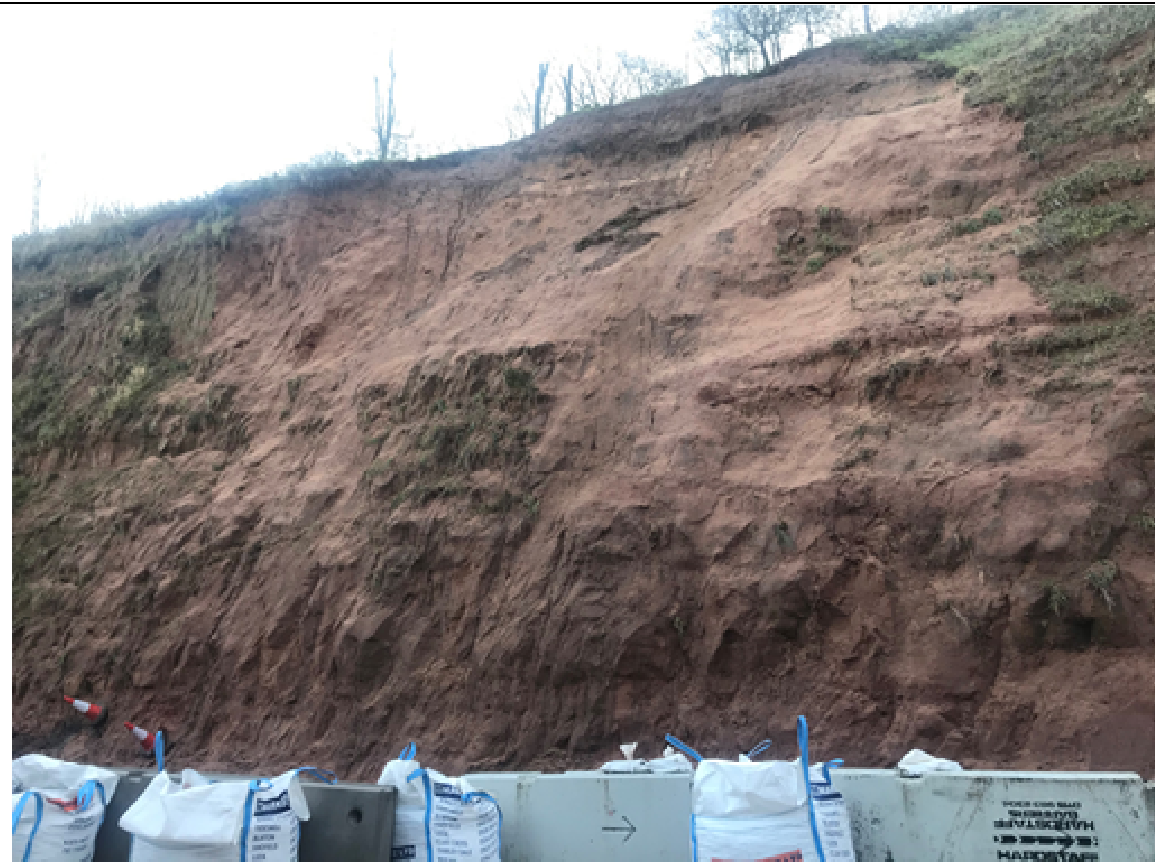
Photograph 2: Previous failure scar (Image taken on 16/12/2019)
