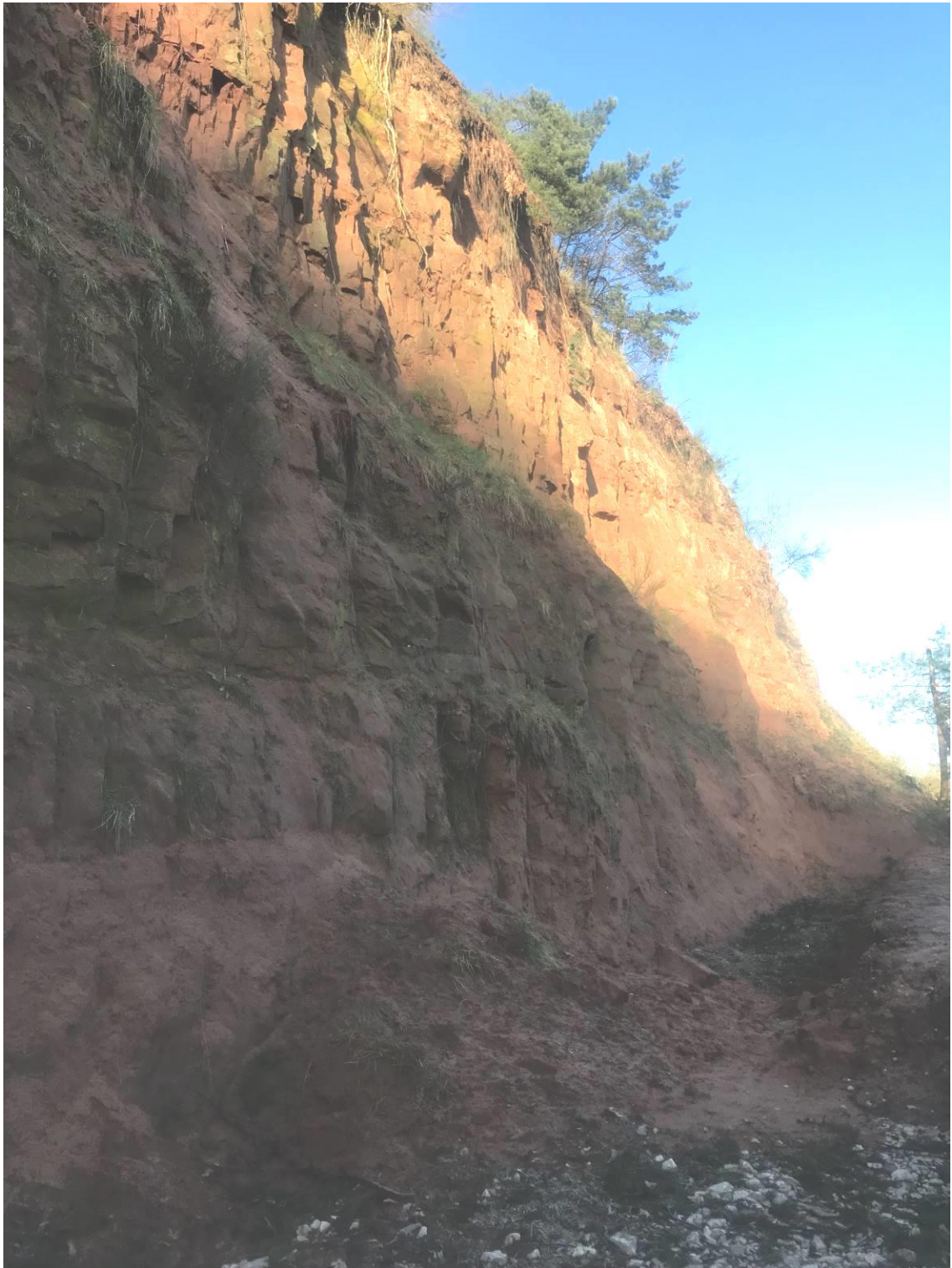
Photograph 5: Looking north to the end of Unit 8. Debris from small failure reported on the 24 th November 2019. Note two grass clumps, approx. 30cm 2 on top of the previous small failure (Image taken on 06/02/2020).
