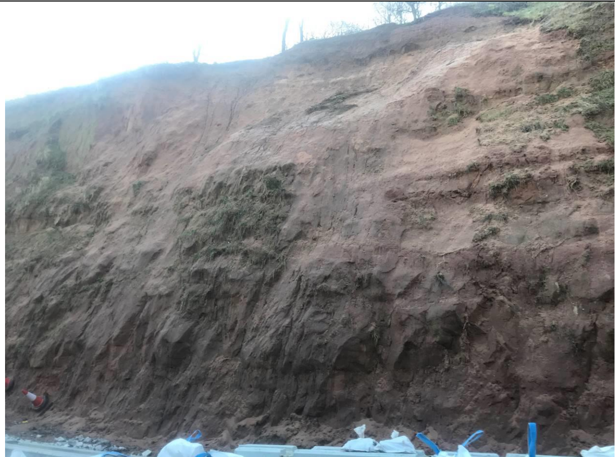
Photograph 2: Previous failure scar (Image taken on 06/02/2020)
